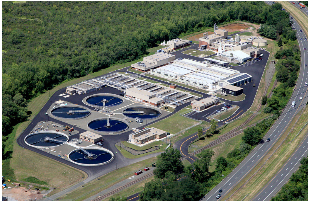
Mattabasett District Water Pollution Control Facility
